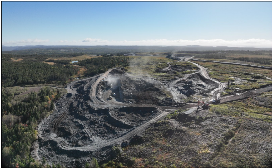
Figure 2. Hammerdown Mine Site – Establishing Initial Mine Benches
